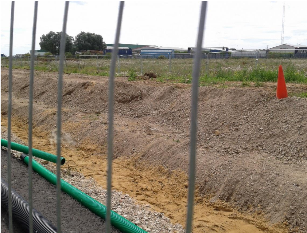
Plate A11.1.1.2 A Culvert is Currently being Installed along the Track in Boston 2
