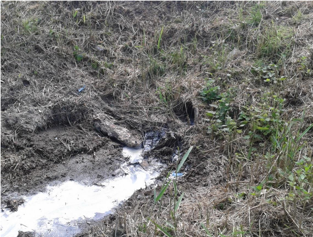
Plate A11.1.1.3 A Partially Collapsed Culver Outfall in Boston 4
